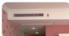
Front air flow, bottom air intake
