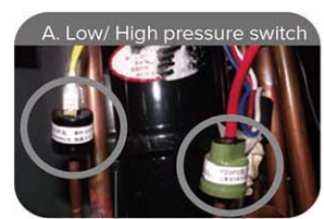
Low pressure switch High pressure switch
