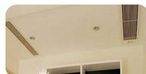
Front air flow, back air intake
